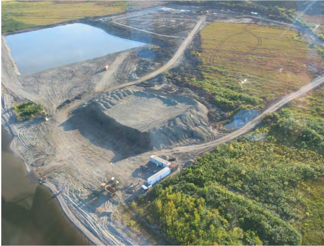
FIGURE 7 - MATERIAL SITE AT NIMIUK POINT
