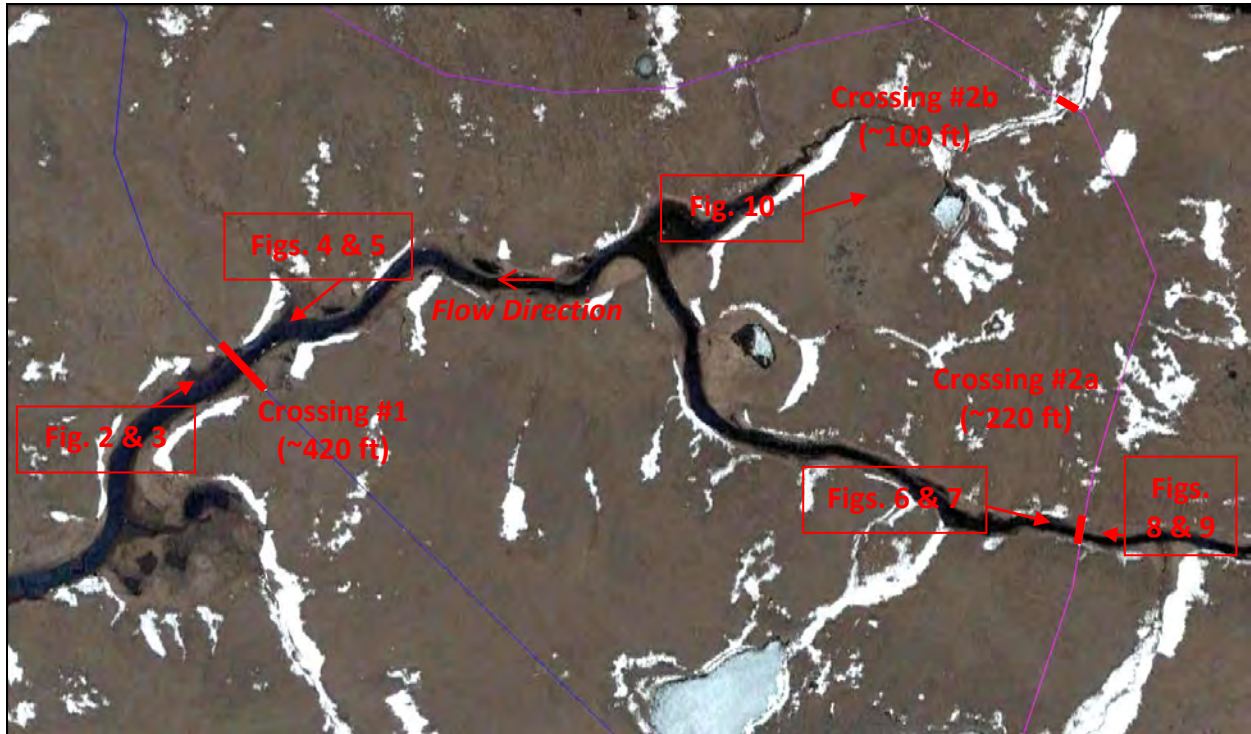
FIGURE 1. An aerial view of Sadie Creek and the stream crossing locations being considered. The straight line distance between Crossings #1 & #2a is about 1.21 miles. (Photo from Google Earth)
