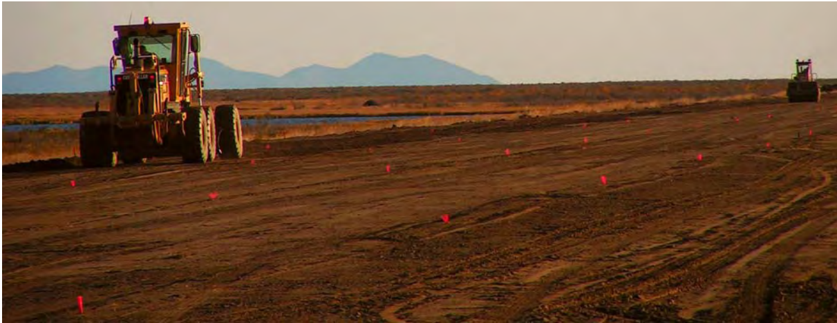
FIGURE 10 - CONSTRUCTION OF A SILT EMBANKMENT AT ALAKANUK AIRPORT (SEPT. 2008)
