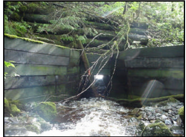
Figure 21 - Auke Nu Creek entering culvert under Glacier Highway
