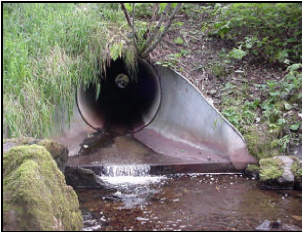
Figure 14 - Bay Creek exiting culvert under Glacier Highway
