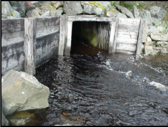
Figure 22 – Auke Nu Creek exiting culvert under Glacier Highway
