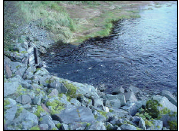
Figure 23 – Auke Nu Creek exiting culvert under Glacier Highway
