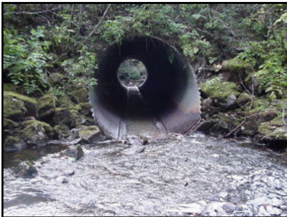
Figure 18 – Waydelich Creek entering culvert under Glacier Highway
