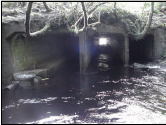
Figure 8 – Auke Creek entering structure under Glacier Highway
