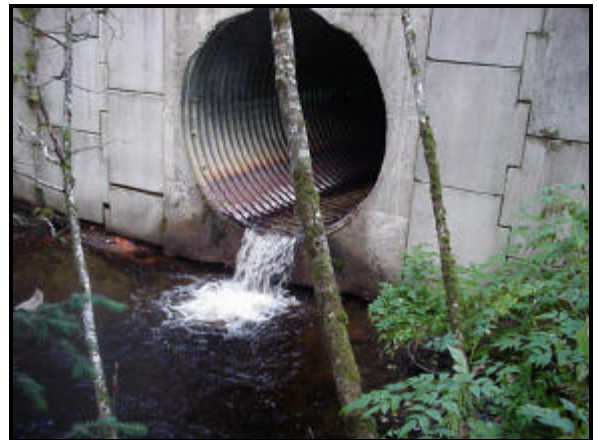
Figure 19 – Waydelich Creek exiting culvert under Glacier Highway
