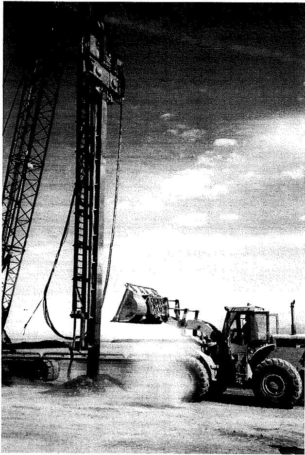
FIGURE 2 – Vibracompaction probe
