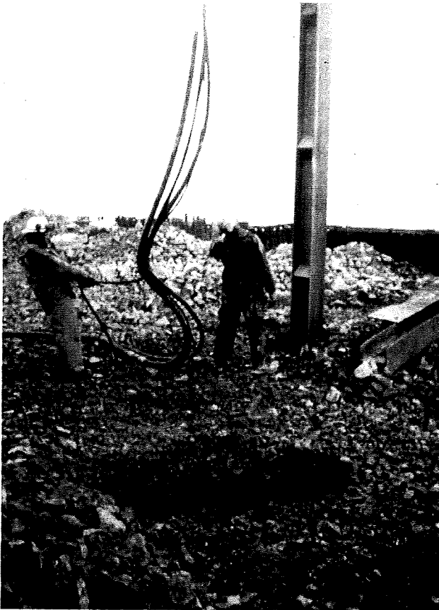
FIGURE 5 – Vibracompaction of shot rock fill at Dutch Harbor, Alaska.
